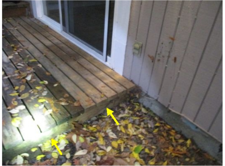
Wood to ground contact at rear deck
