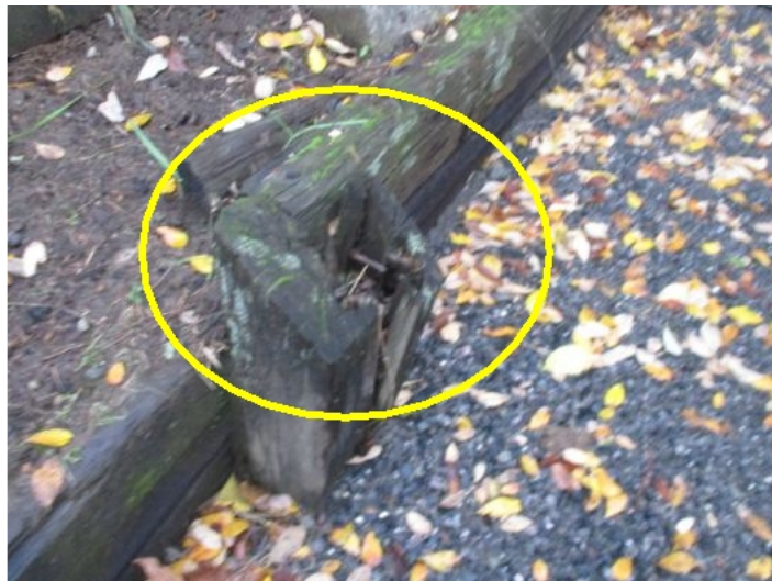
Rotted post at left retaining wall
