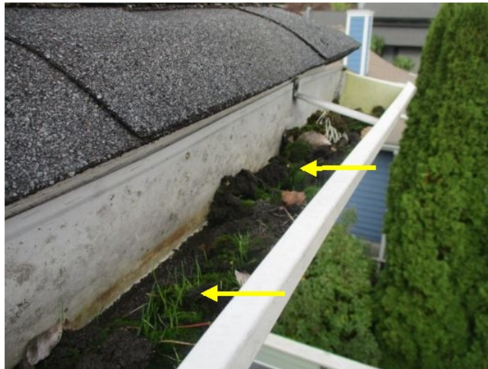
Observed gutters full of organic debris
