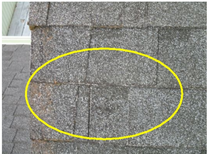
Granular loss on shingles
