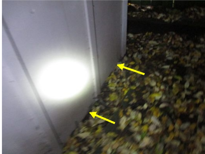
Wood to ground contact at shed siding
