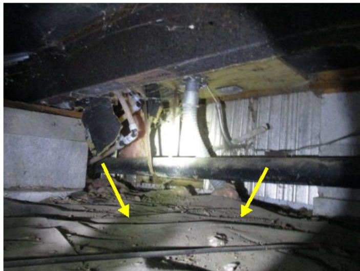
Exposed soil in crawl space
