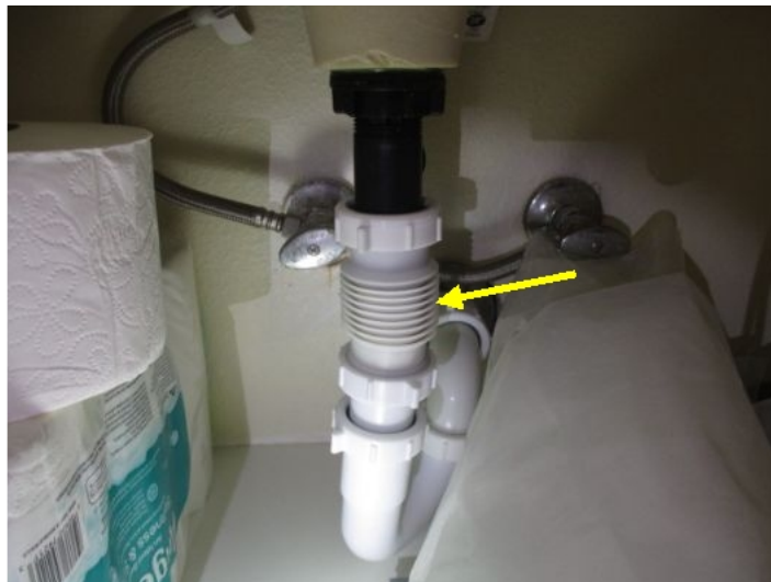
Flex style drain pipe in south bathroom
