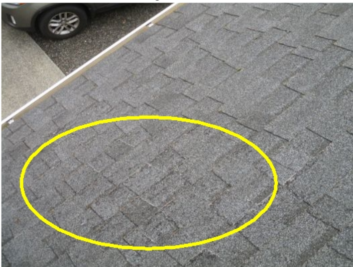
Granular loss on shingles
