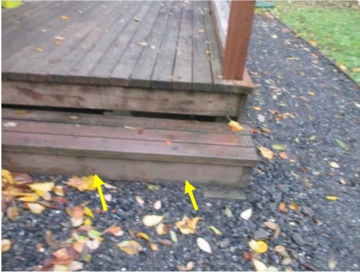
Wood to ground contact at front deck
